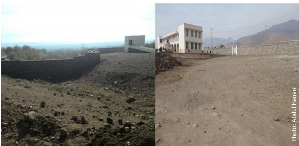
Gulbahar number one high school before and after rehabilitation
